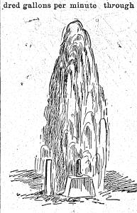
NIOBRARA'S ARTESIAN WELL. eight-inch pipe, and with a pressur of ninety-five pounds to the square inch the water rises to an elevation of eighty feet. The spectacle as the jet shoots upward and breaks and falls in masses of spray is one of great beauty. The water has a temperature of seventy degrees. The well is owned by the milling company of the enterprising town.
