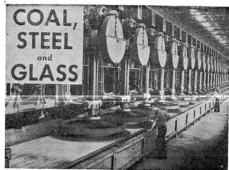
Polishing plate glass in Pennsylvania factory
