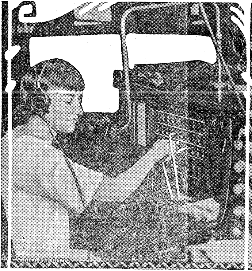
Elsie Turnbull, blind since her eighth birthday, at work on the five-trunk board which she operates most efficiently for a large firm of St. Louis, Mo. It was difficult for her at first, but six months made her very efficient. The five trunk lines coming into the board are equipped with bells of different tones so that she can distinguish them by sound. The sixteen inside stations are also known to Miss Turnbull by sound.
