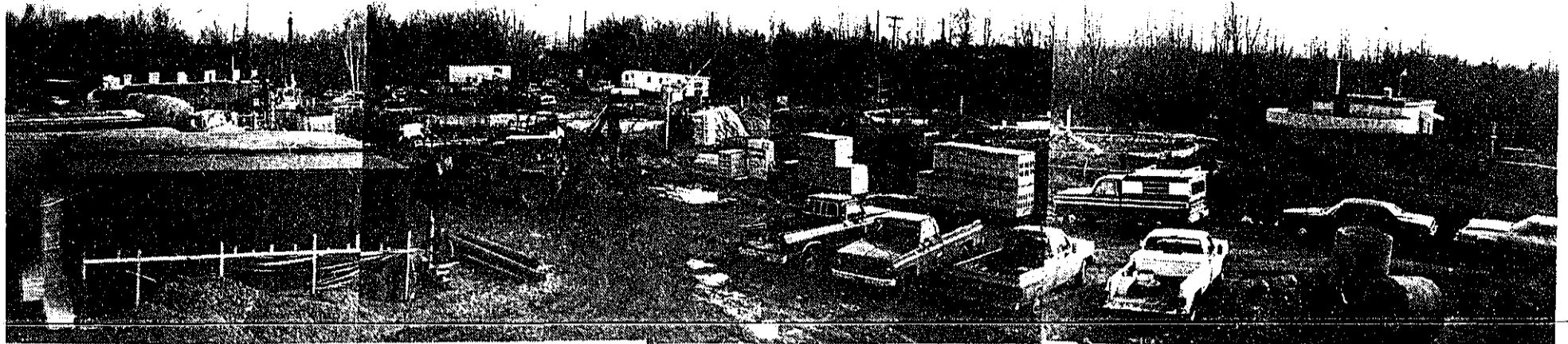
OVERALL VIEW of the $6 million Cass City wastewater treatment plant expansion project. Work is being done on several parts at once, ranging from the control building at left, behind trailers, bio-disc structure behind the tractor and two new secondary settlement tanks, behind the present plant at right.
