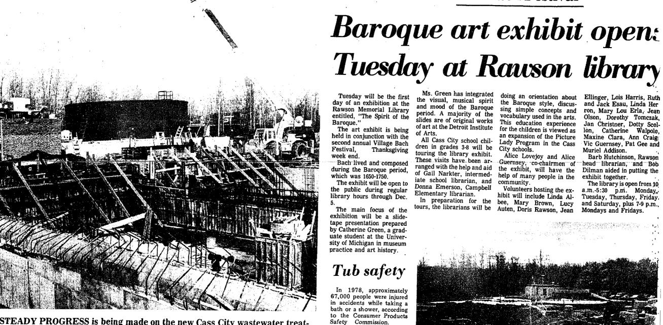
STEADY PROGRESS is being made on the new Cass City wastewater treatment plant expansion and improvement project. In the foreground is the structure that will contain the bio-discs to decompose bacteria; at left is a portion of the control building, and the large tank in the background will be the equalization basin.
