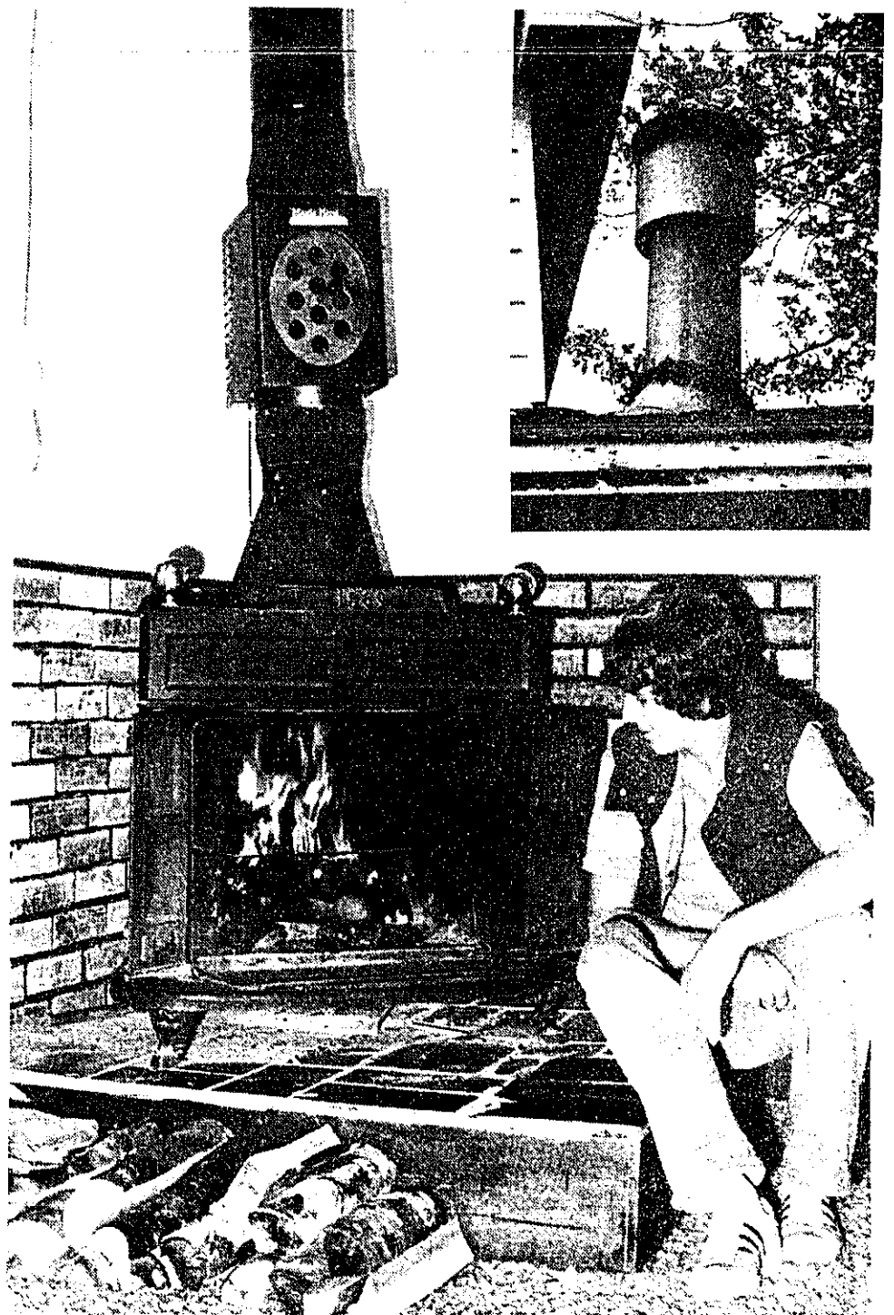
ENJOYING THE HEAT from the Franklin wood burning stove in the home of Elkland Township Fire Chief Jack Hartwick is son Rob. The stove is elevated off the floor, sits on slate, is a safe distance from the walls, which are covered with fireproof imitation brick. The smokestack (inset) as it goes through the roof is surrounded by two larger pipes.
