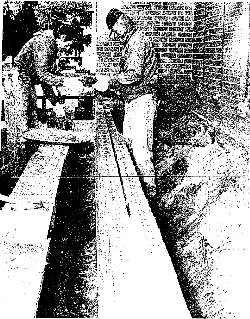
NEW FLOWER BOXES in front of Rawson Memorial Library are being built by George Lynch (left) and Wayne Dewey. The old ones had deteriorated and would have eventually fallen down. The masons will complete the new ones this week.
