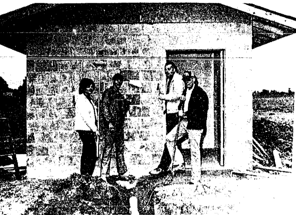
RESTROOMS -- It was too wet Friday to get any work done, but among those building the restrooms at the Owen-Gage football field are volunteers, from left, Sandy Peters, Danny Ondrajka, Robert McPhail and Dick Glidden.
