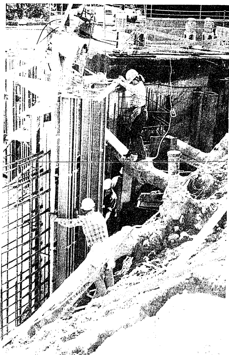
SECONDARY TANK -- These workers are guiding a form into place for pouring of concrete for one of the two 42½-foot in diameter secondary settling tanks. At top right is apprentice carpenter, Cecelia Kartes, the first woman member of the 360-member Bay City Local 116 of the Carpenters Union. (Another photo page 1.)
