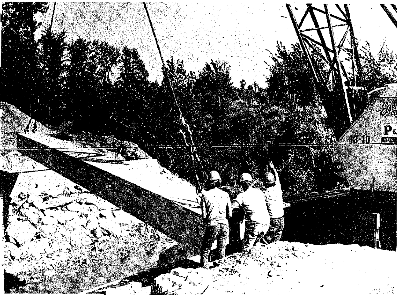
BRIDGING THE GAP-- Beams for the Deckerville Road bridge over Mud Creek, east of Cemetery Road, were installed Friday. The bridge may be open in about a month. Eisenhour Construction Co. of East Lansing is the contractor, with the approximately $75,000 project being paid for with 80 percent federal funds, 10 percent state and 10 percent from the Tuscola County Road Commission.
