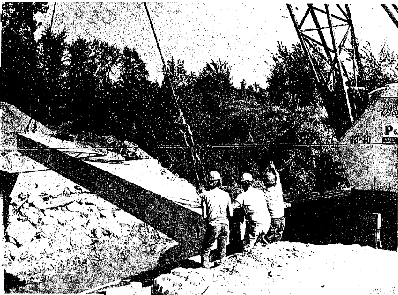
BRIDGING THE GAP -- Beams for the Deckerville Road bridge over Mud Creek, east of Cemetery Road, were installed Friday. The bridge may be open in about a month. Eisenhour Construction Co. of East Lansing is the contractor, with the approximately $75,000 project being paid for with 80 percent federal funds, 10 percent state and 10 percent from the Tuscola County Road Commission.
