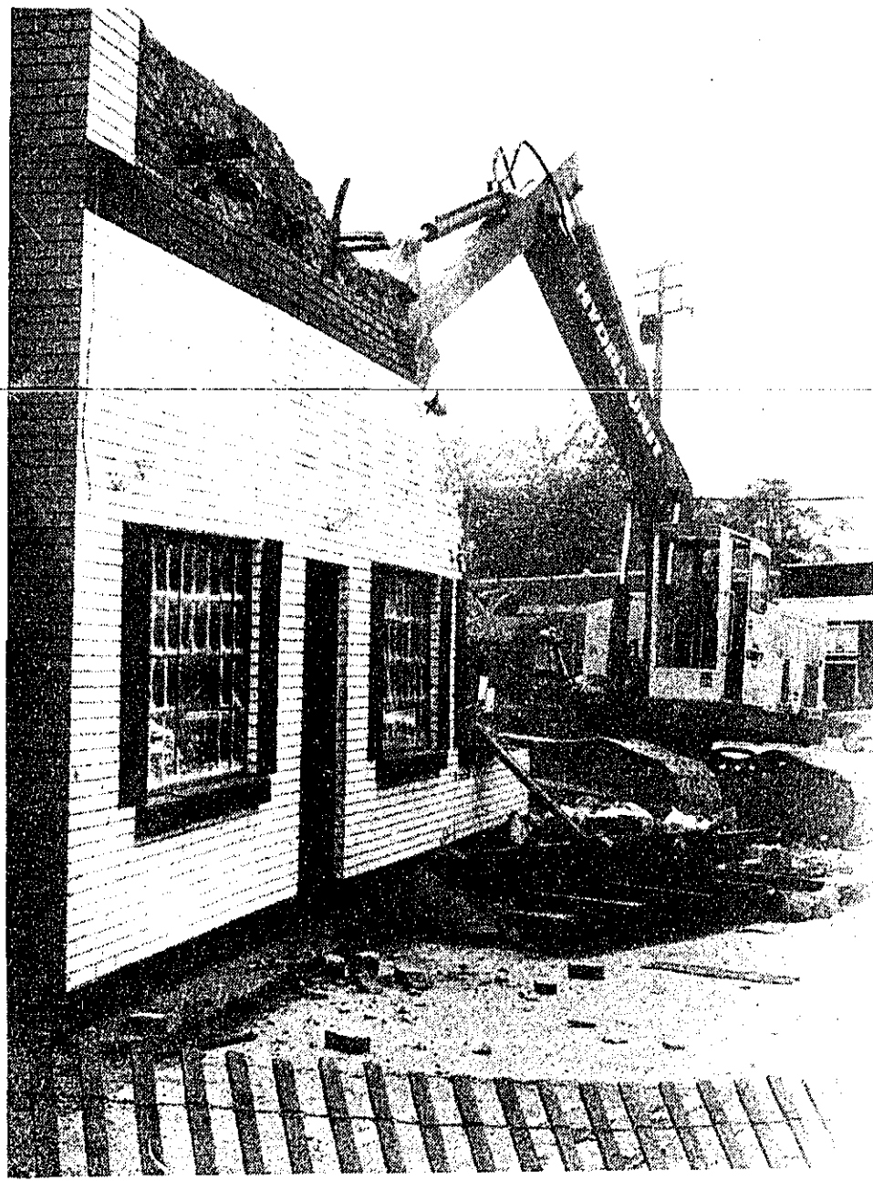
NO MORE GAS -- The S T & H service station which had stood at the southeast corner of Main and Seeger Streets since about 1928 was demolished Monday. The Pinney State Bank next door has purchased the property, according to Fred Pinney, but plans for its use are still indefinite. Rooney Contracting Co. of Bad Axe did the demolition.
