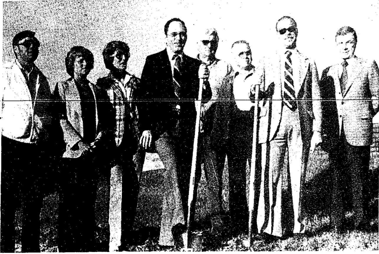
BREAKING GROUND -- On hand for the groundbreaking of the new waste water treatment plant are, from left, council members Elwyn Helwig, Lynda McIntosh, Dorothy Stahlbaum, village superintendent Lou LaPonsie, plant supervisor Nelson Willy, Dick Hampshire, village president Lambert Althaver and Delbert Rawson. Before the ceremony Tuesday morning the council met to approve the plant's operating budget and loan resolution.
