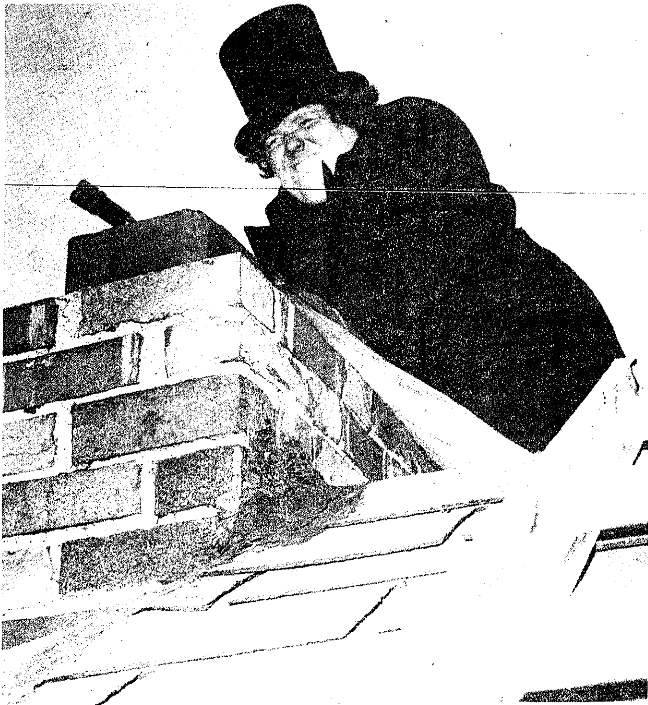
CLEANING CHIMNEYS is hard work, as evidenced by the grimace on Irene Ferguson's face. The rods in the canvas bag, protruding over the side of the chimney, are attached in sections to the wire cleaning brush. The Pigeon resident was cleaning the chimney of Mr. and Mrs. Lloyd Frederick, of Evergreen township. (Story on page 18.)
