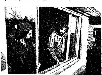
SAVE HEAT by replacing old, worn-out windows with pre-fin-ished, aluminum-framed, thermalized ones such as this tripleslider being set into repaired window frames. Other aluminum replacements can be fitted to any size or shape window. All come in a wide variety of baked-on colors, are maintenance-free, lightweight and easy to handle. If your prime windows are still good, add aluminum storm windows for ex-
