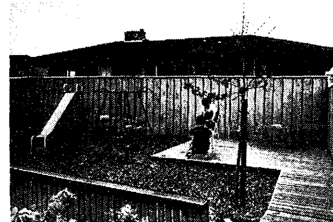
ROOM TO RUN without trampling the garden is provided by play area enclosed by fences of 1x6-inch western wood along property lines. Lower fences inside the yard are of 1x2s on 2x4 stringers. Decking of 2x4-inch Douglas Fir and wood chips on ground reduce weeds, dust and mud.
