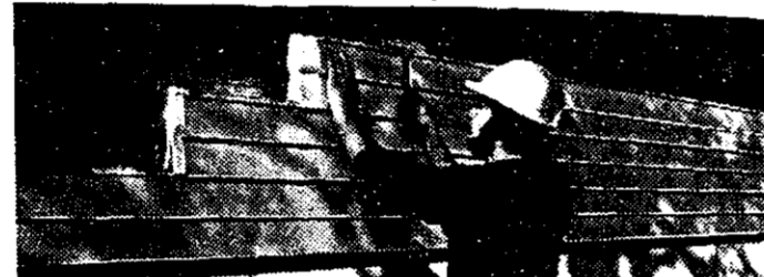
INSULATED ALUMINUM SIDING can make you more comfortable and help you conserve energy. It comes in factory-laminated backer board, as drop-in inserts placed behind the aluminum siding, or in panels installed under the new siding.
