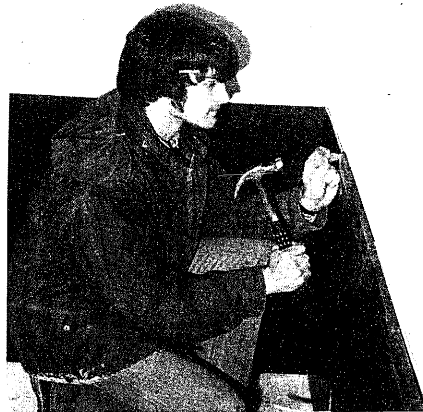
INSIDE -- Rob Clarke nails on the edging of the half-paneling in one of the bedrooms. All of the walls have new plasterboard. The small house has two bedrooms, bathroom, kitchen-dining room and half basement.
