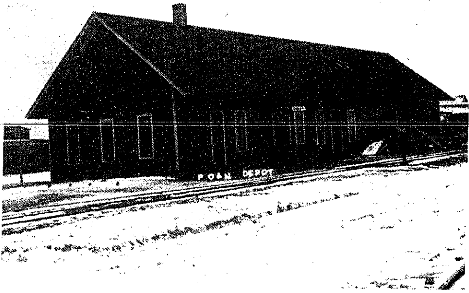
ORIGINAL DEPOT? -- This may have been the original Pontiac, Oxford and Northern depot in Cass City. Meredith Auten believes it burned down.
