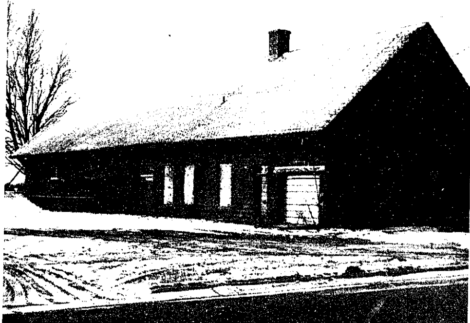
FINAL DAYS -- The present depot at Garfield and Vulcan Streets, soon to be torn down, was apparently built in 1907.
