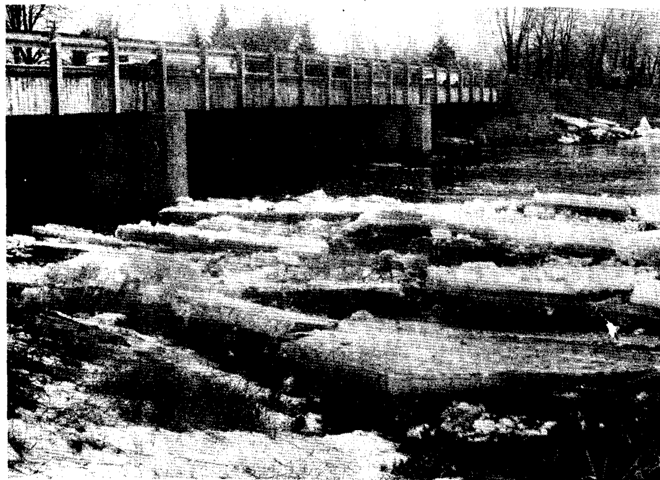
ICE JAM - These large chunks of ice almost totally blocked the south span of the Cemetery Road bridge over the Cass River Monday. Due to the rapidly melting snow over the week end, the rapidly flowing river was several feet higher than normal.
