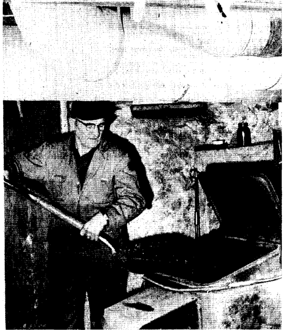
STOKING UP — Peter Zell dumps a shovel full of coal into the stoker, which automatically feeds it into the furnace. The stoker normally feeds coal for one minute every half hour. It only has to be filled once a day.
