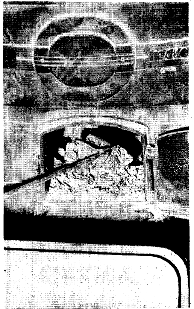
TONGS are used to remove the "clinkers" from inside the burner. Sometimes, but not in this instance, they are still glowing.
