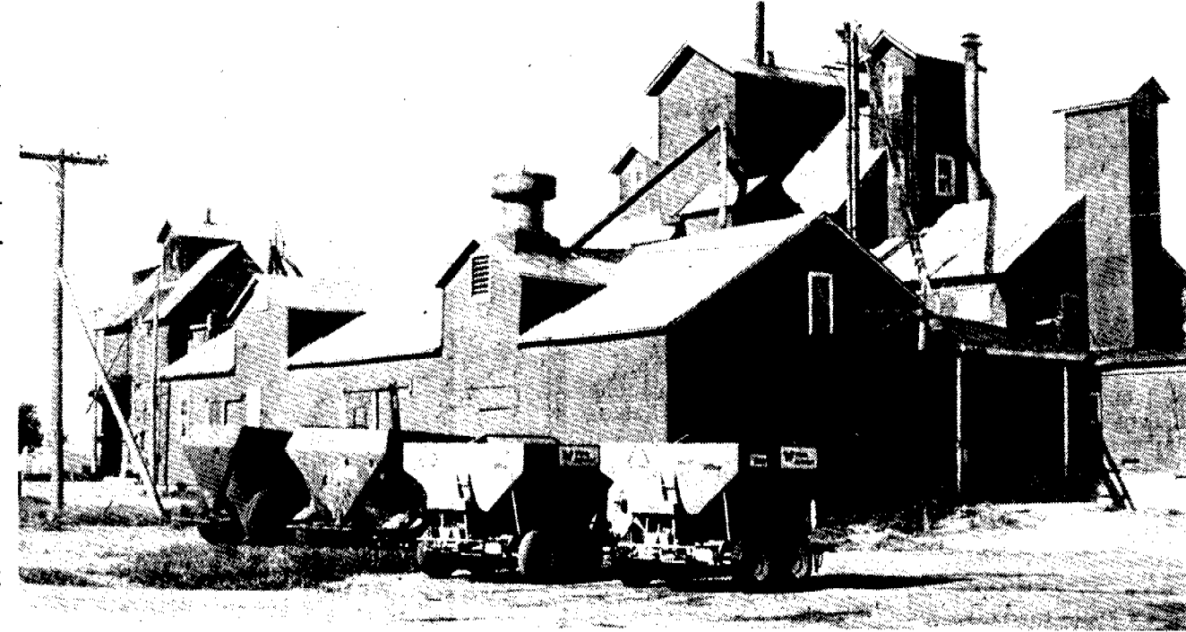
WAITING FOR DEMOLITION -- The two elevators are still standing, with demolition tentatively scheduled to start some time this winter. Photo was taken this summer, when Wickes Agriculture was still using the site for some purposes.
