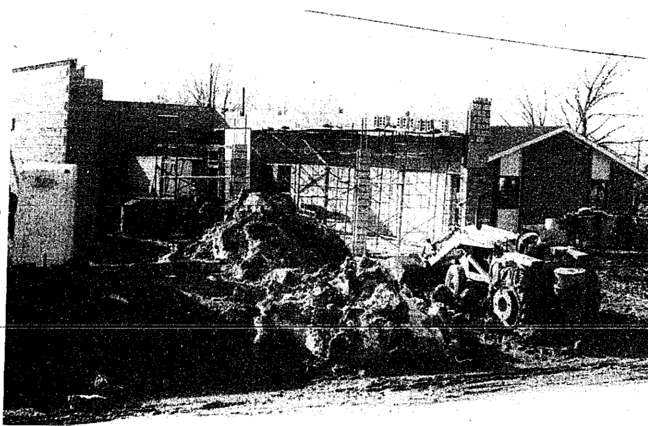
TOWNSHIP - VILLAGE HALL - Work on the Elmwood township - Gageton village hall and fire station is proceeding, with construction scheduled to be completed this summer. Booms Construction Co. of Bad Axe is building the $173,000 building. Federal public works funds are paying $150,000 of the cost; the village and township are splitting the remainder.
