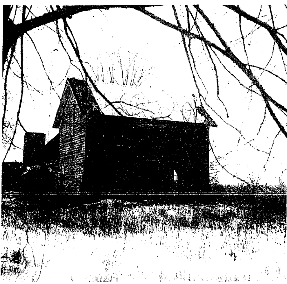
ABANDONED -- Snow and an abandoned home on Cemetery Road, south of Cass City, created this winter scene.
