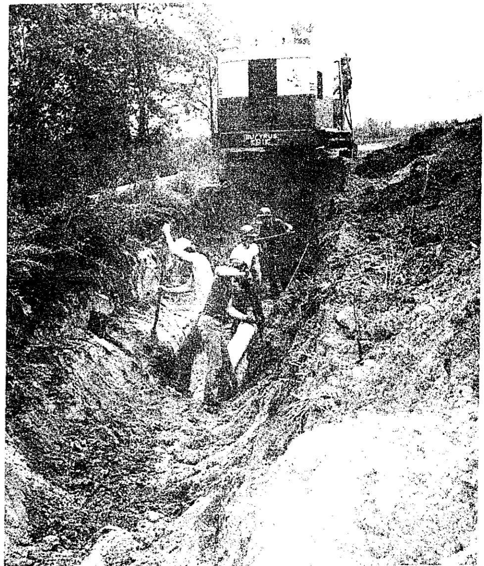
DIGGING IN -- Workmen from the Andrew Barnes Construction Co. have been busy installing water and sewer lines in the Cass City industrial park in the southwest corner of the village. Work on the project is expected to be completed in about two weeks. Cost is $39,571, plus engineering fees and other expenses.
