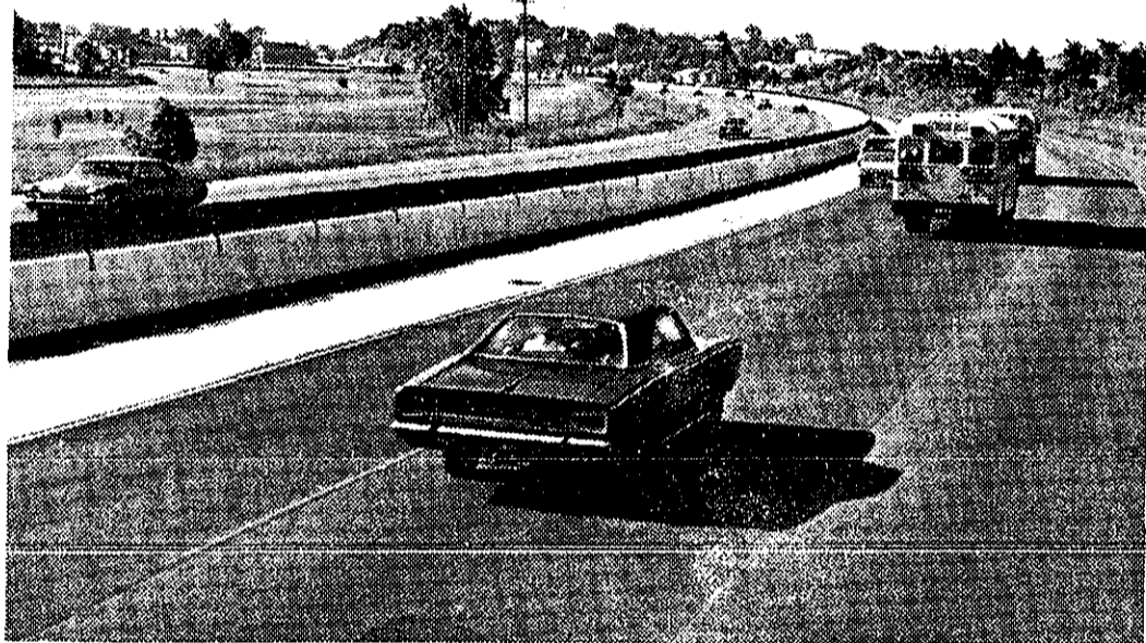
NEW BARRIERS FOR SAFER DRIVING—Concrete median barriers like this one on I-75 west of Flint have replaced metal guardrails on more than 100 miles of urban freeways in Michigan. Topped by concrete or metal head-light glare screens, they're shaped to direct wayward vehicles back into the travel lane.
