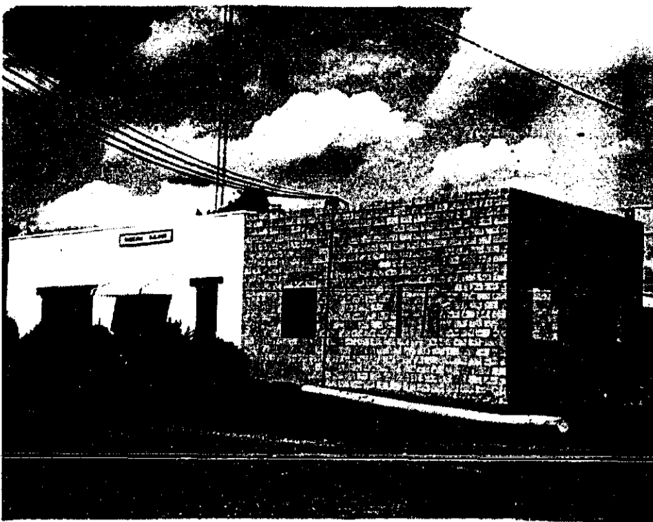
THINGS ARE changing at Cass City's municipal building. Work is progressing on a 23 by 28-foot addition that will provide much-needed office space. The addition will cost about $12,000. Another $6,000 will be spent on an addition to the village garage.
