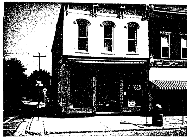
LARGE STORE BUILDING with about 1600 feet on first floor, large 3 bedroom apartment upstairs, full basement with oil furnace, corner location, located in the heart of town. If you want to get into business look this one over. Asking $18,000.
