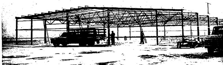
Cuckler rigid frames for excellent strength and roof loadings to meet today's construction standards.
