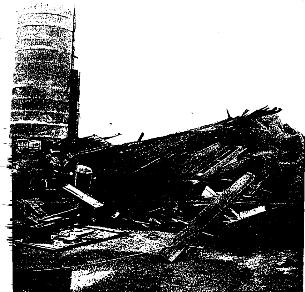
HIGH WINDS demolished a 30 by 70 foot barn belonging to Harold Polega located on Bay City-Forestville Road east of M-53. Lost were a steer, 200 chickens and several ducks. Machinery stored in the barn was also damaged when the building collapsed.
