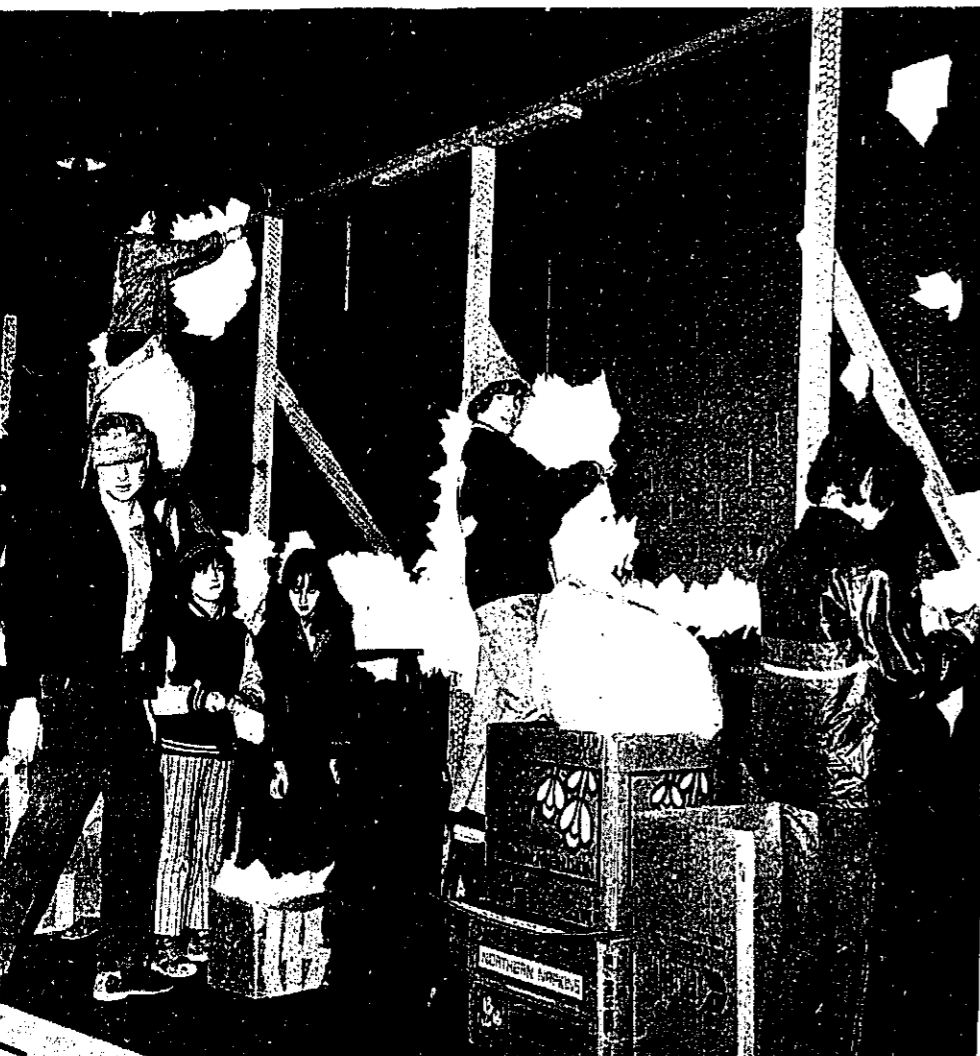
THE GIANT SIGN placed at the corner of Main and Seeger was built by volunteers Tuesday.
