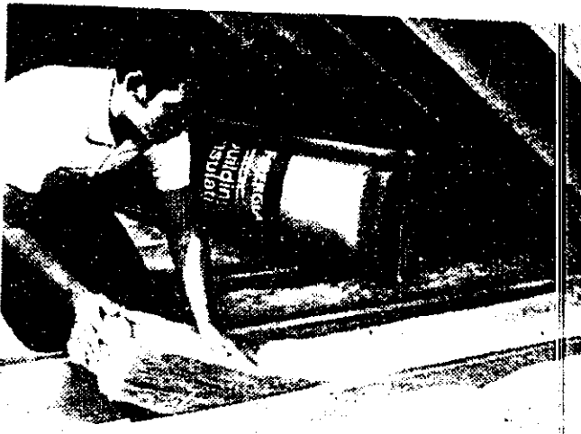
INCREASED ATTIC INSULATION CAN conserve heat and cut fuel bills. Blankets of insulation six inches thick provide optimum performance, and can be installed by the homeowner.
