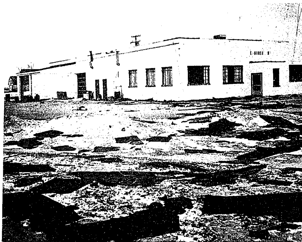
THE GALE WINDS Saturday afternoon caused thousands of dollars worth of damage in the Cass City area. Television antennas, roofs, trees and small buildings tumbled before the wind's blast. Among the hardest hit was the engineering building at Walbro Corporation. The roof was literally lifted from the building. Workers said that you could stand in the building and look up to the sky Monday morning. Some of the pieces of the roof are visible in this picture. Other pieces stretched for 300 yards and more.
