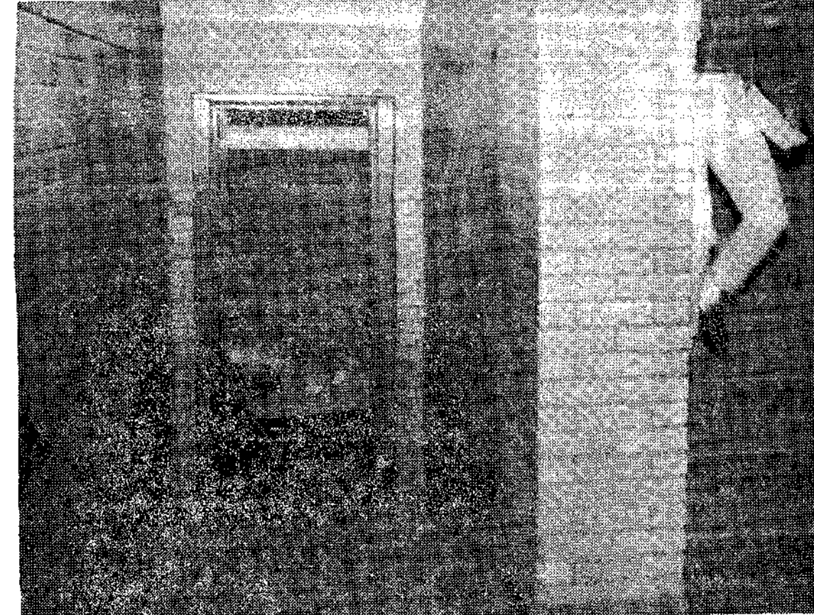
THROUGH THIS DOOR and under the steps at the right is the Cass City High School sick room where ailing students are kept until they can be taken home or given treatment. The tiny cubicle, listed as inadequate at a recent public meeting on the proposed new high school, contains a cot, a chair and a sink. (Chronicle photo)
