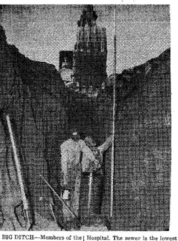
in the village. The extreme depth Cass City maintenance crew are dwarfed by the 17-foot ditch was made necessary because the hospital site is on a hill. (Photo dug last week for the sewer to by Neitzel, engraving courtesy the new Cass City Community of Bay City Times.)
