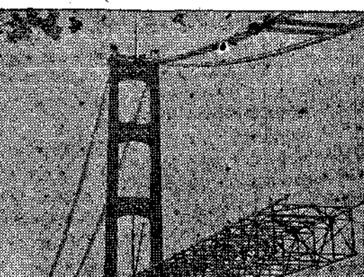
Just inches to go and this stiffening truss unit will take its permanent place in the huge Mackinac Bridge. More than sixty per cent completed, this phase of the work will be finished by American Bridge in the latter part of July.
