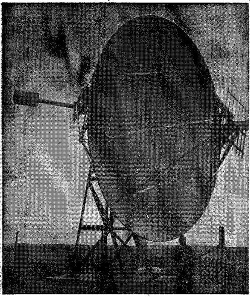
**BIG EAR**—University of Michigan astronomers and electrical engineers have set up this 28-foot-wide radiotelescope near Ann Arbor to receive radio signals from the sun. The sensitive device is expected to be in operation in February, providing information about the sun's outer atmosphere. The work is being supported by the Office of Naval Research through the University's Engineering Research Institute.
