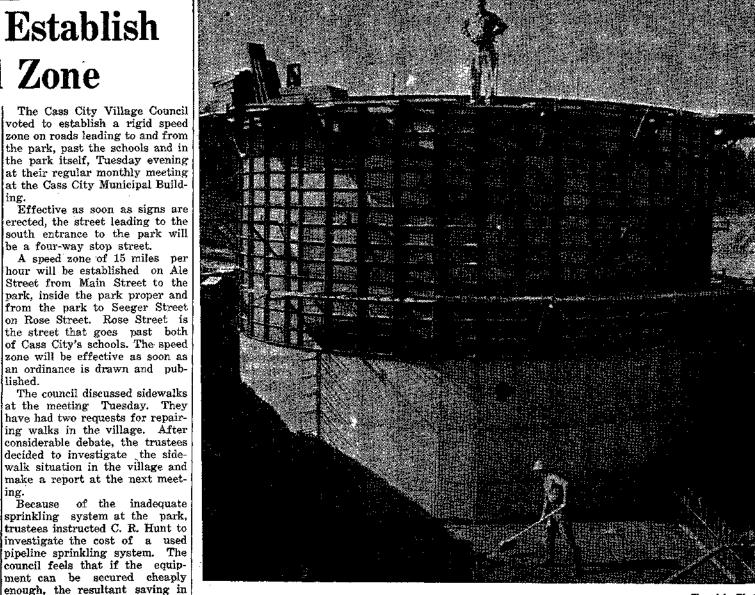
MAKING PROGRESS-Work on the addition to the sewage disposal plant in Cass City is proceeding on schedule, according to persons in charge of its construction. The big tank is the digester which is expected to eliminate the village's disposal problems. The pit in the foreground will house the controls and a building will also be erected at this spot. Work on the project is expected to extend into the winter months. The village hopes to have the plant in operation in January, 1956.
