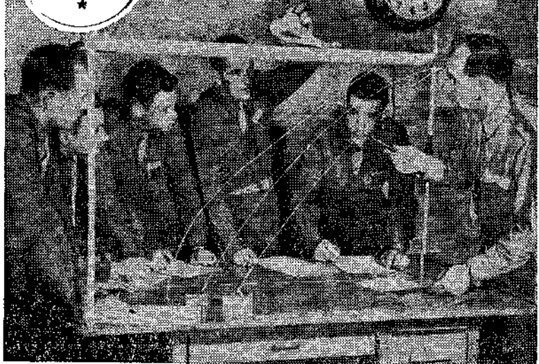
Synthetic trainer. Miniature plane slides along track at top, releasing toy bombs along wire tangents.
