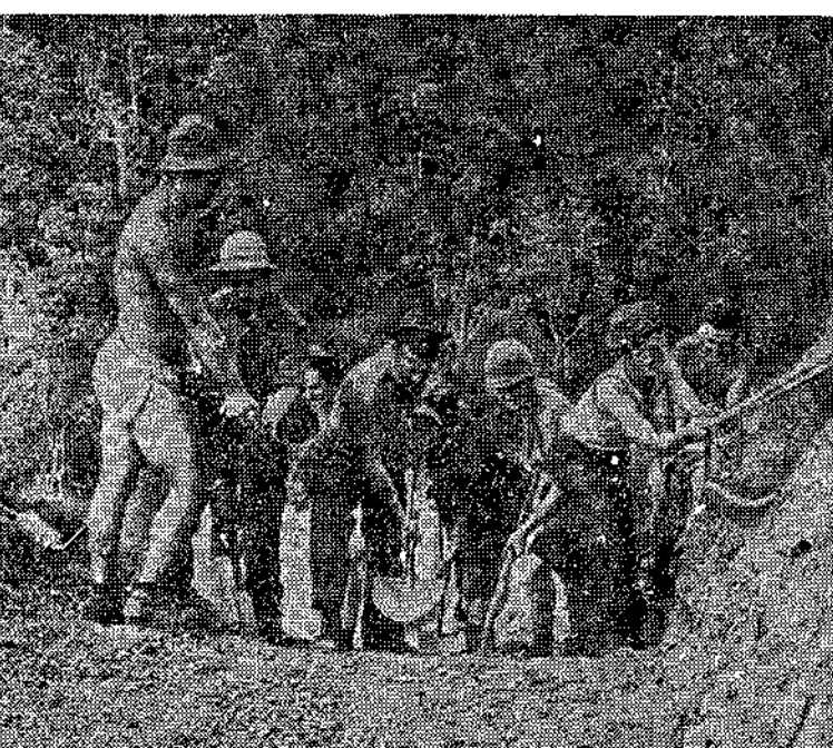
Building "Pee" roads in New Guinea is all part of the day's work for American army engineers. This particular road under construction near Port Moresby, main Allied base in New Guinea, is so steep that the men must hold on to ropes to keep from falling backward. The grade drops about 65 degrees behind them.
