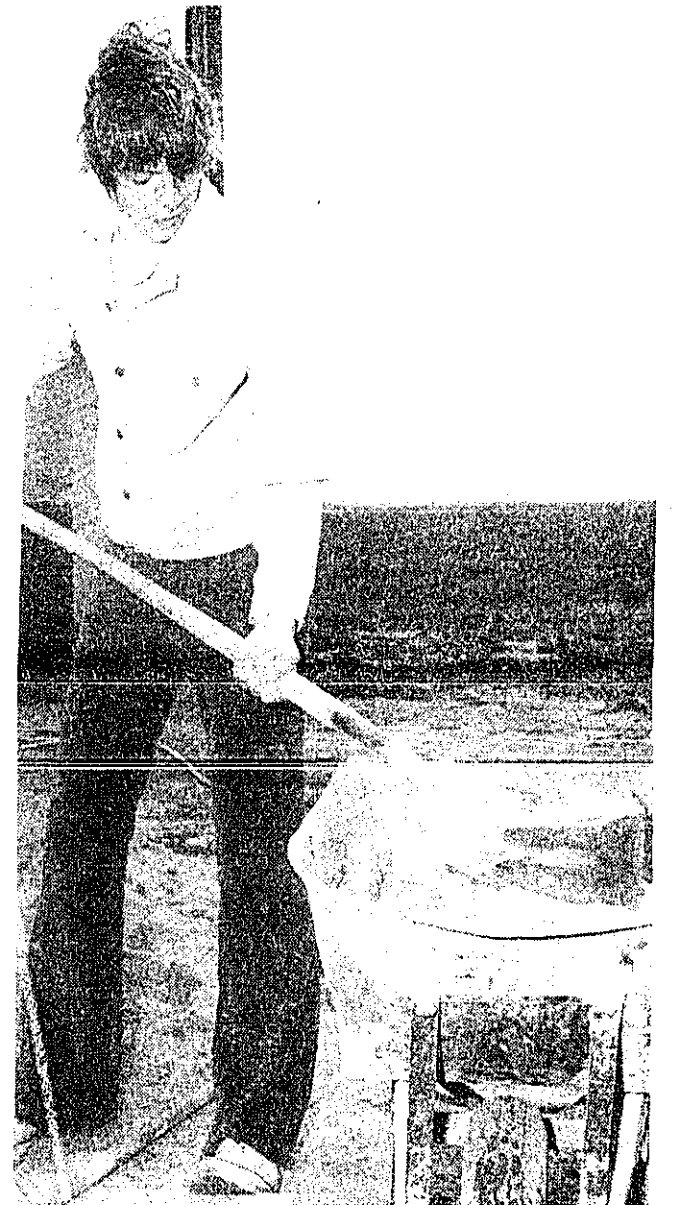
MIXING CEMENT takes just the right combination of ingredients as Owen-Gage student Aaron DeMorrow is learning. He's one of about 20 students helping construct new dugouts at the school's athletic field.
