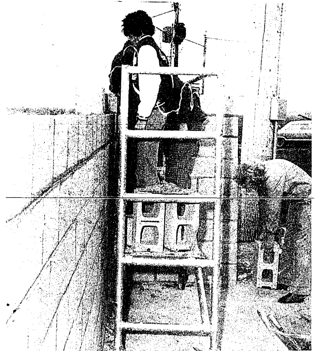
THESE OWEN-GAGE students are learning masonry first-hand as they help construct new dugouts at the school's athletic field. The project is one phase of field renovation that included a recently-constructed cinder track.
