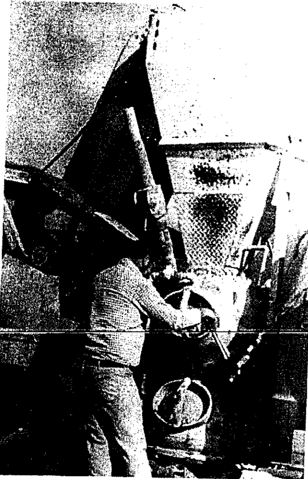
FROM THIS mixer the liquid cement goes into the hose, visible at bottom of picture, and then to the construction site 50 feet or more away.
