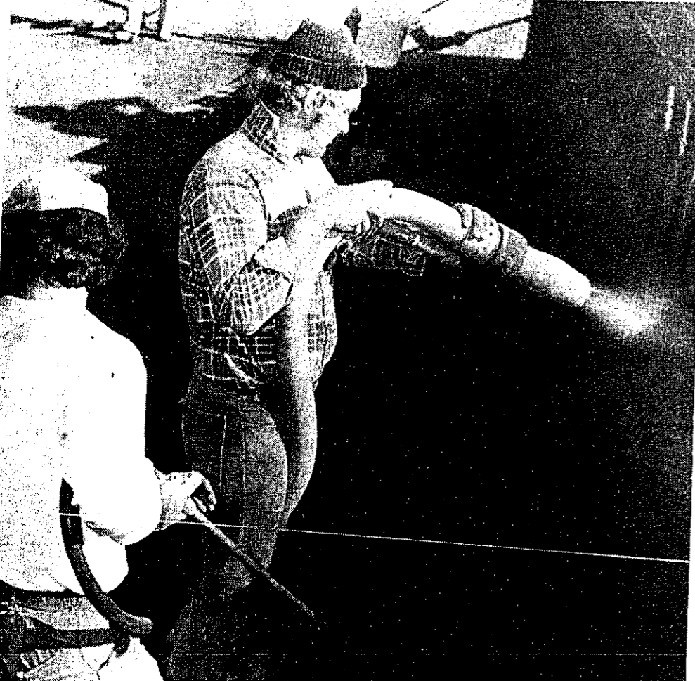
THIS IS THE WAY the cement for the new swimming pool is "poured". The system is quick. Eighty 94-pound bags of cement per hour go on the wall of the pool. The entire job will take an estimated 1,100 bags.
