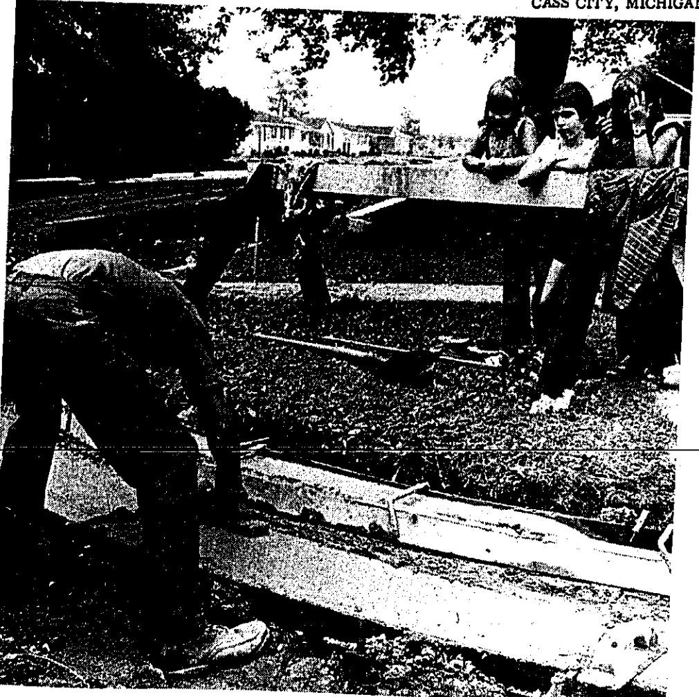
SIDEWALK SUPERINTENDENTS come in all sizes and ages. Here, (from the left) Andrea Nieboer, 8, Lynn Weippert, 5, and Andrea's twin sister, Angela, look on intently as Andrew Barnes puts the finishing touches on a section of curb and gutter at the corner of Third and Woodland Streets.
