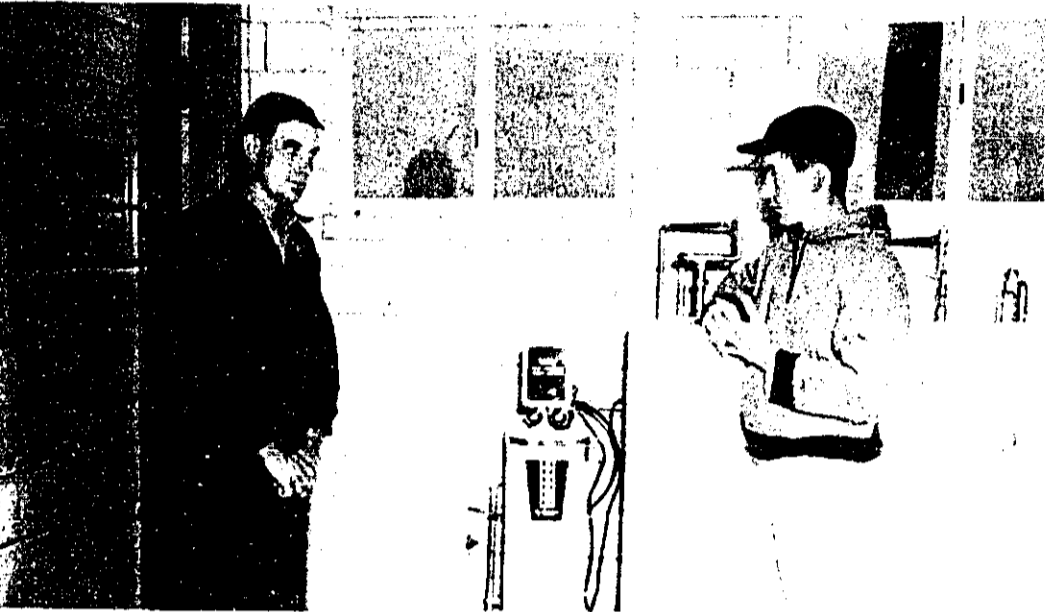
WATER USED TO CLEAN the equipment in the Loomis dairy barn is prepared with water softening equipment, shown here. According to Dave, at right, soft water requires less soap than hard H2O.
