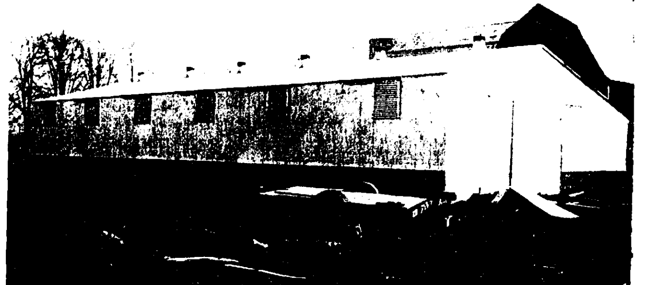
The above picture is the new beef barn 50' x 100' offset open side for outside feeding, on the Eugene Foote Farm, 1 mile east of Argyle.
