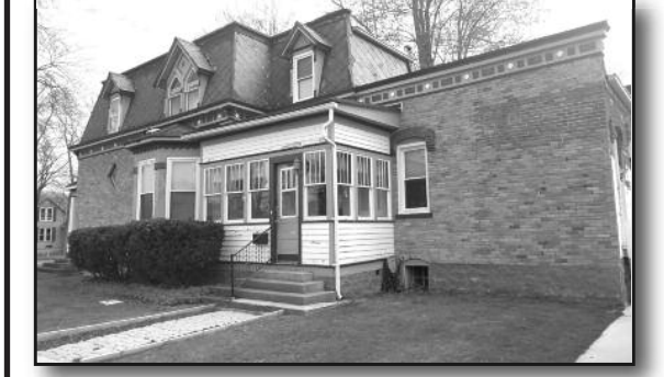
4243 Seeger St. Cass City $99,000 Beautiful historic 4 bed, 2 bath home with many updates including plumbing & electrical. Includes a heated 24' x 48' shed.
