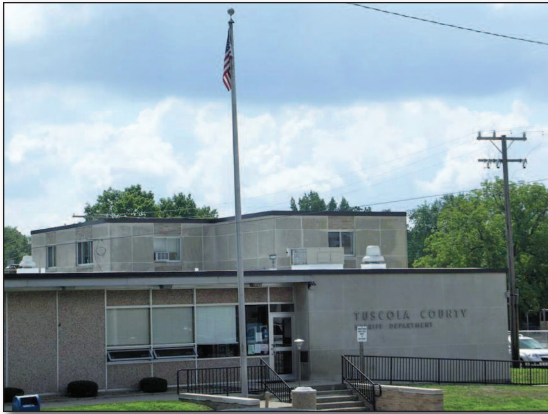
THE MAIN part of the Tuscola County Jail at 420 Court Street, Caro, was built in 1966 and has since undergone several renovations. A recent study of the facility shows it is outdated and a new jail should be constructed.
