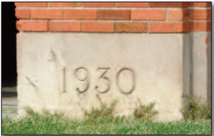
A SECTION of the school that was built in 1930 will be demolished, but the plan is to try to save the cornerstone, which might have a time capsule buried behind it.
