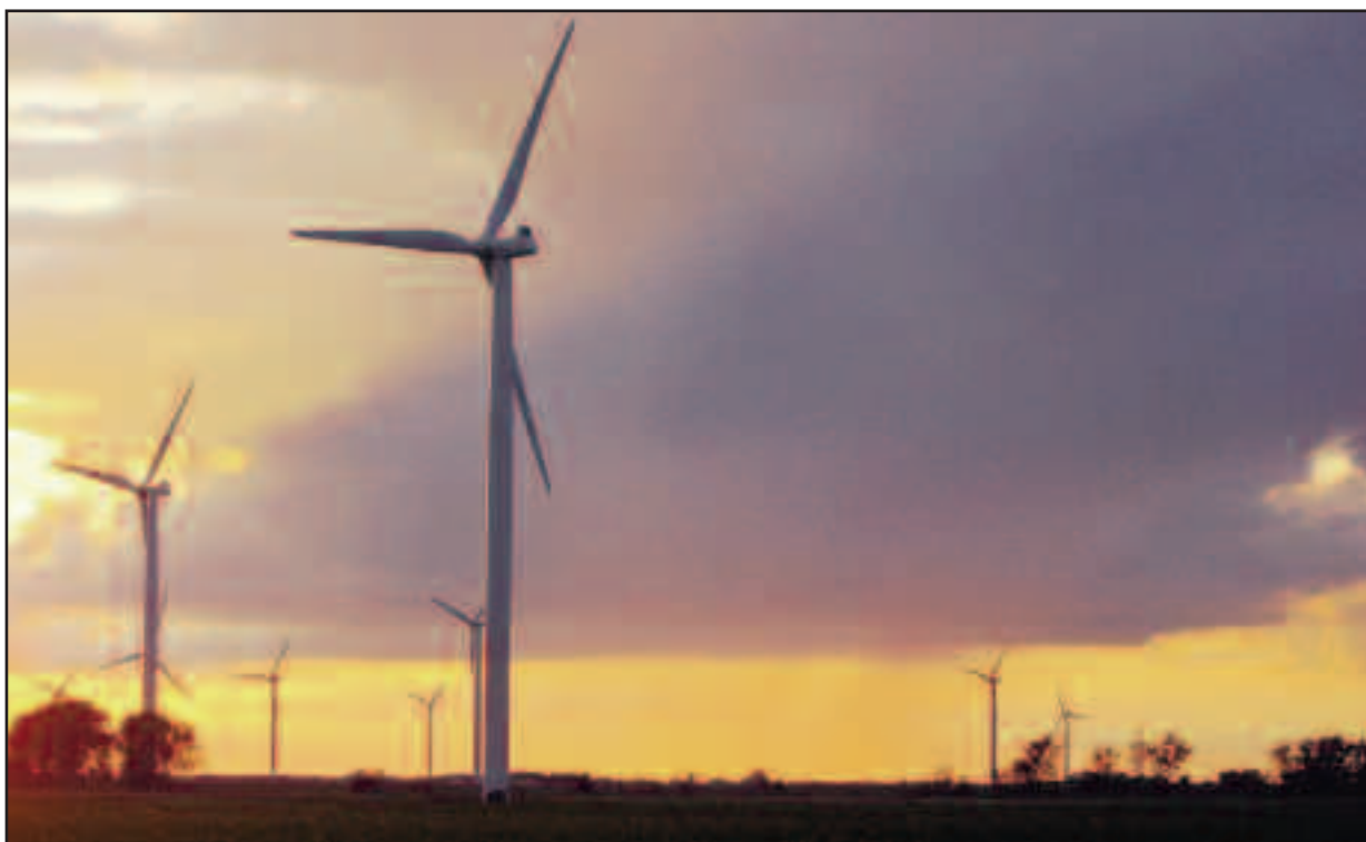
NEXTERA ENERGY Resources is in the process of developing Tuscola III Wind Energy Center in Almer, Ellington and Fairgrove townships. When completed, the project will add 52 turbines to the skyline in those townships. (Mary Drier photo)
