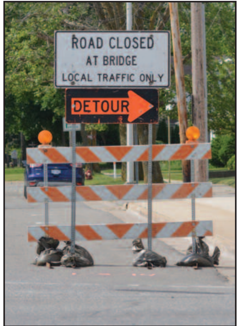
SIGN OF THE TIMES. The Tuscola County Road Commission began an estimated 5-month construction project Monday to replace the Cemetery Road Bridge.
