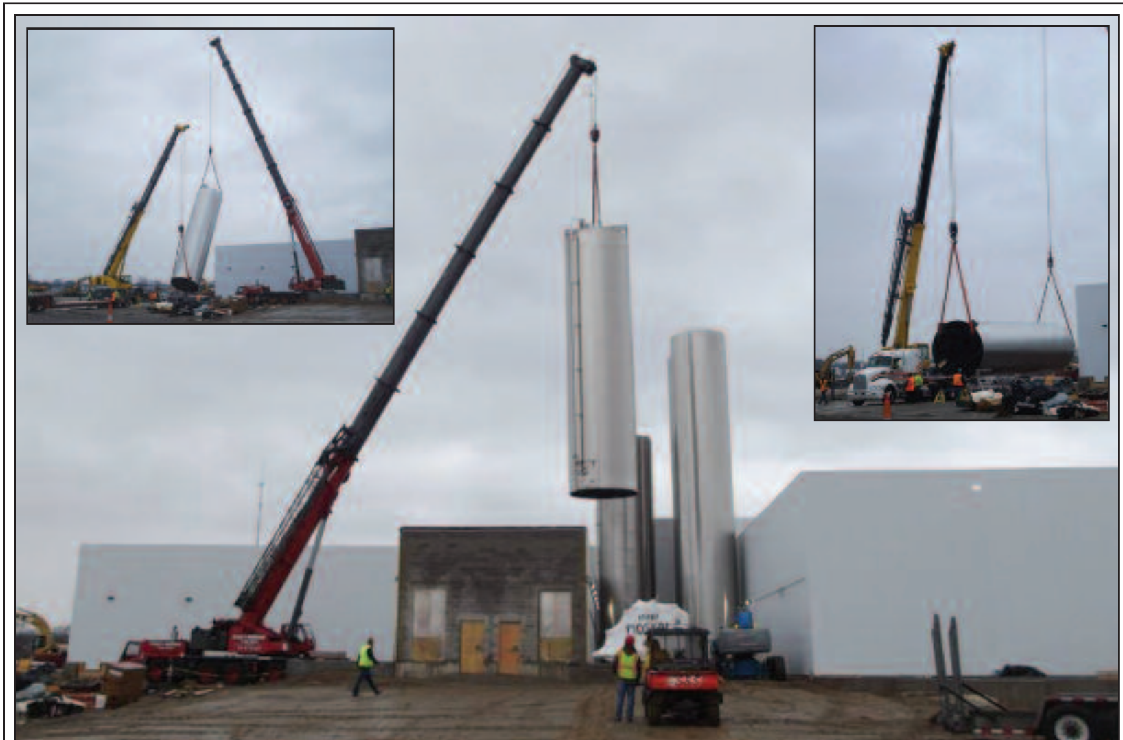
CONSTRUCTION CREWS continue to make steady progress on the new Dairy Farmers of America (DFA) milk processing plant, located in the Cass City Industrial Park. Above, crews set a 40,000-gallon silo weighing in at roughly 35,000 pounds. When the construction is completed, there will be a dozen silos with storage capacities ranging from 20,000 to 60,000 gallons. (Photos courtesy of Tyler R. Perry)
