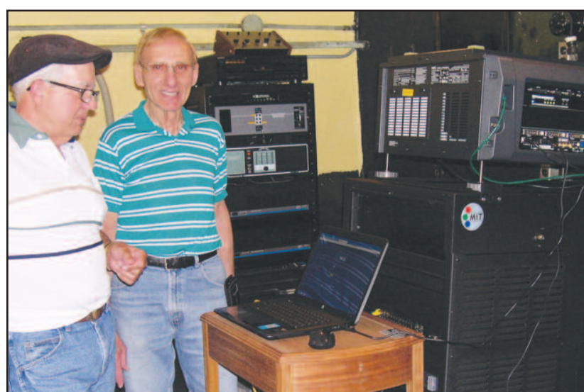
CASS THEATRE owner Dick Hendrick (right) and friend Bob Montgomery work on the new digital projection system now up and running at the Cass Theatre — the Thumb's first theatre to switch to the high-tech equipment.
